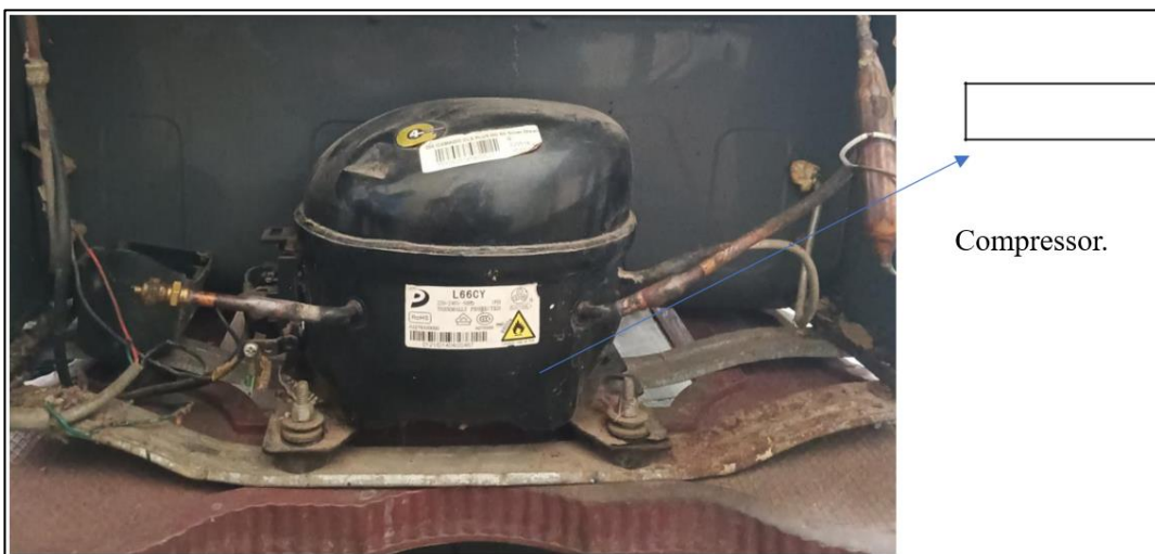
Figure 1.4: Compressor
