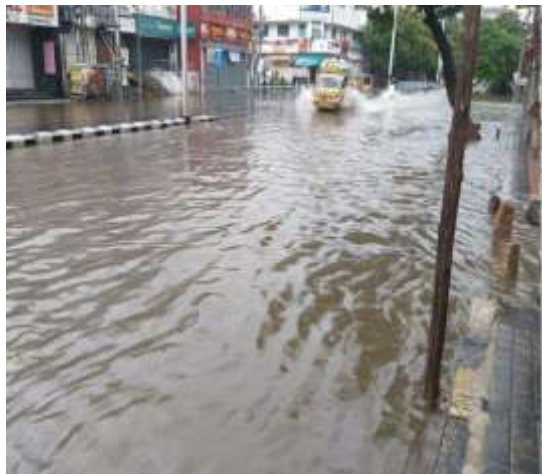
Figure.2.3 Rainwater logging on roads
