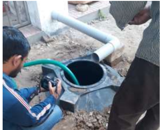
Figure.2.7 Water Storage tank at University Campus
