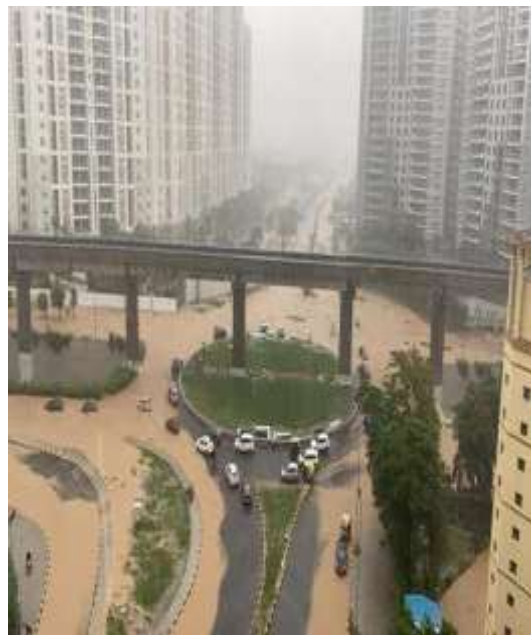
Figure.2.5 Rainwater logging on highways
