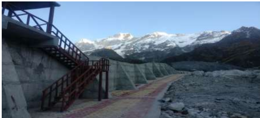
Figure 5.3: a three tier wall-ongoing project in Uttarakhand. [9]
