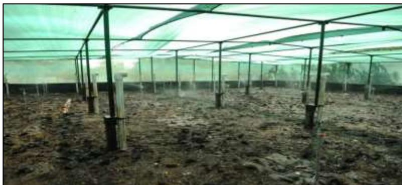
Figure 19.5: Inner View of VERMIFILTER Plant in Gujarat, India with Verm filter Bed & Sprinklers Spraying Sewage over the Soil in Bed inhabited by Earthworms
